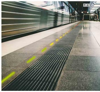
Possible way of indicating free train sections: LED control system from SIUT with colour signals
